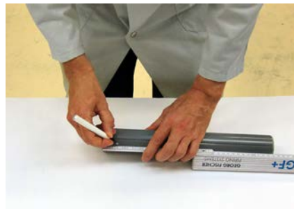
Marking the jointing length
