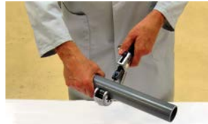
Cutting the pipe to length
