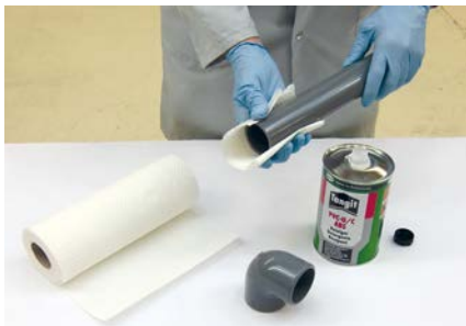
Cleaning the pipe and socket
