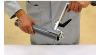
Chamfering the pipe
