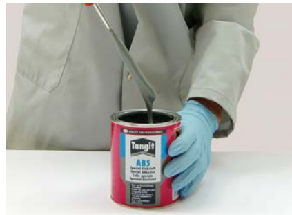
Checking the cement
